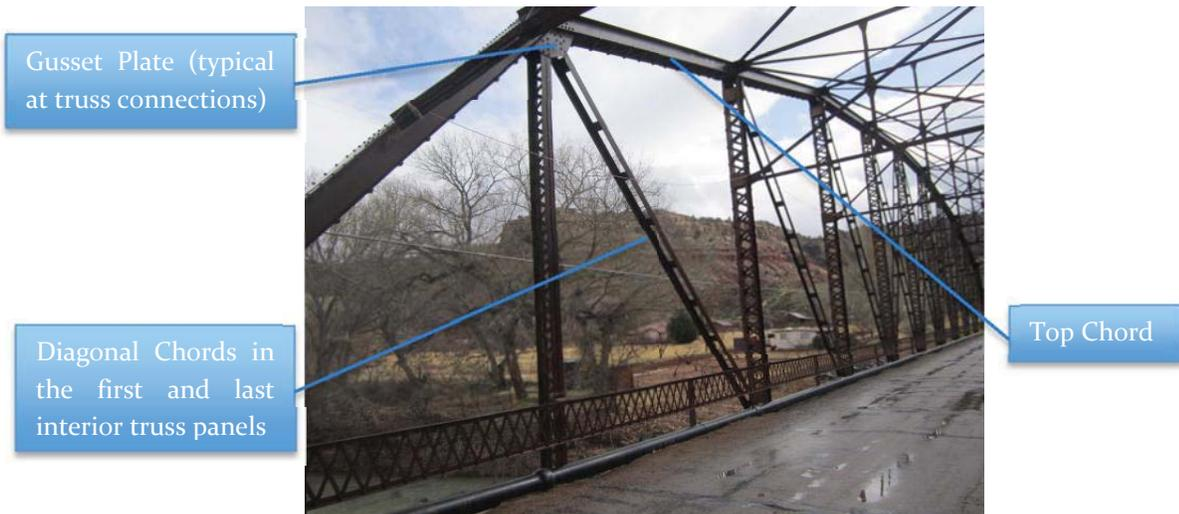
**FIGURE 2 - TRUSS MEMBERS AND CONNECTIONS**
